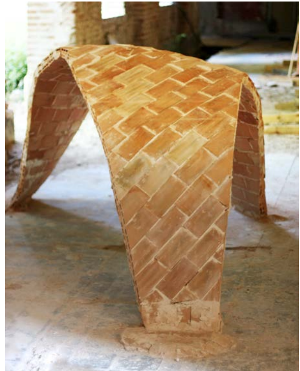
Figure 9. Resulting vault after two layers of tiles.
